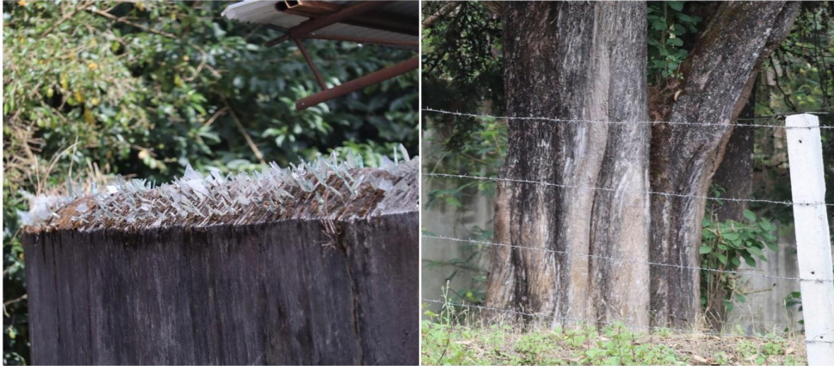
Figure 2. Walls lined with broken glass shards (left) and Barbed wire fencing (right) found near that area.
